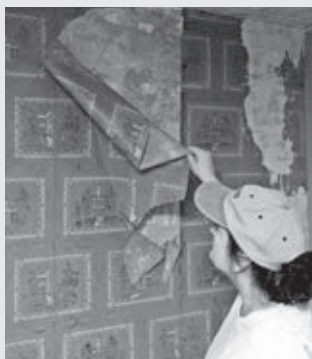
Potentially facing multiple layers of paper, vinyl papers or painted over wallpapers, removal calls for patience and elbow grease more than anything else.
